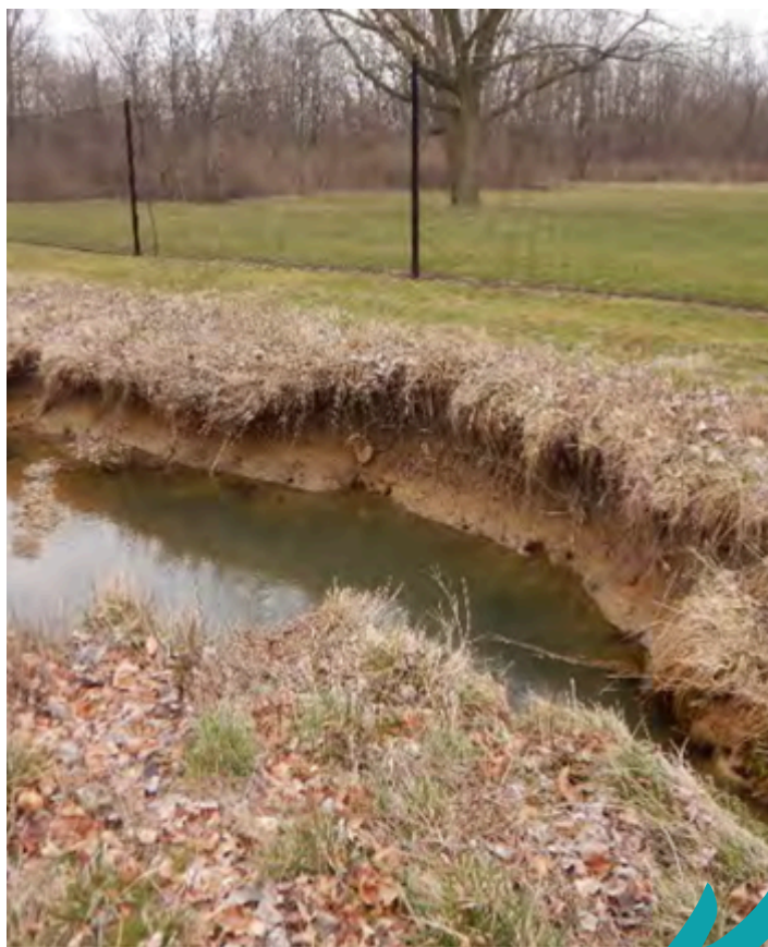
Erosional hot spot along backside of the driving range
